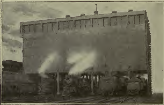
Fig. 78. Electrically Operated 2000-Ton Coaling Station Fourteen engines can be supplied simultaneously with coal, sand, and water. Courtesy of Link-Belt Company, Chicago
